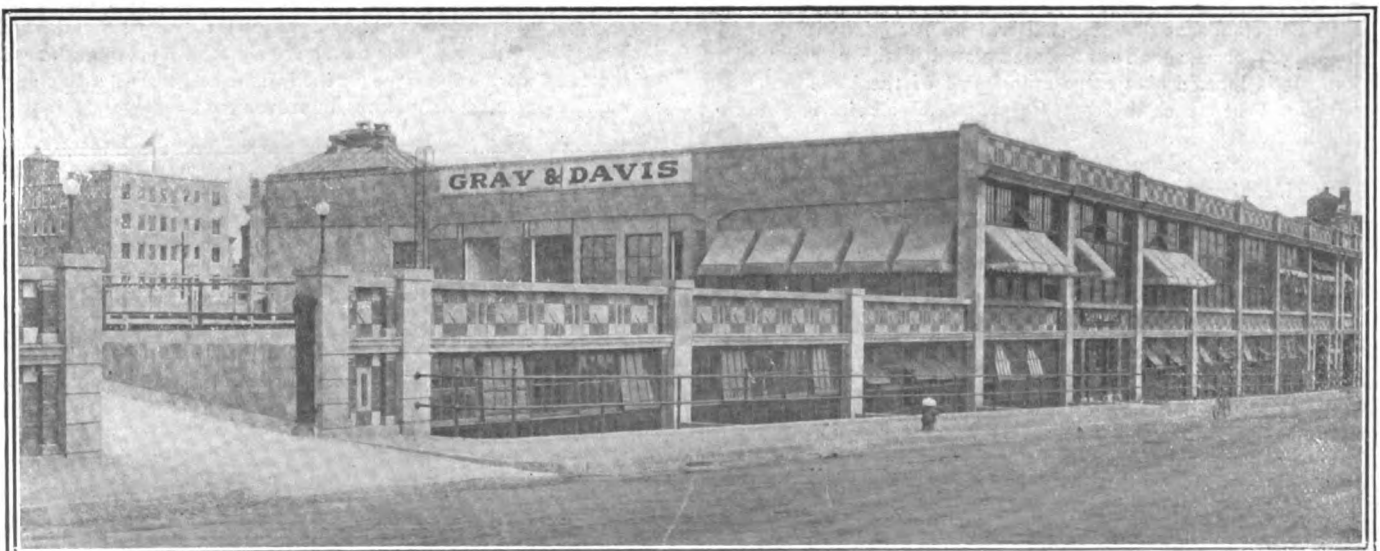
The new Gray & Davis factory building, Boston, which is devoted exclusively to the manufacture of dynamos for use in automobile lighting. The factory is constructed entirely of cement brick
